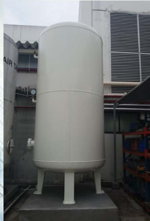
Buffer Tank 10 m 3
