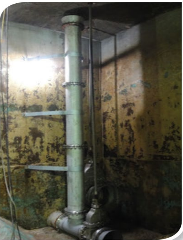
Before installing collecting well
