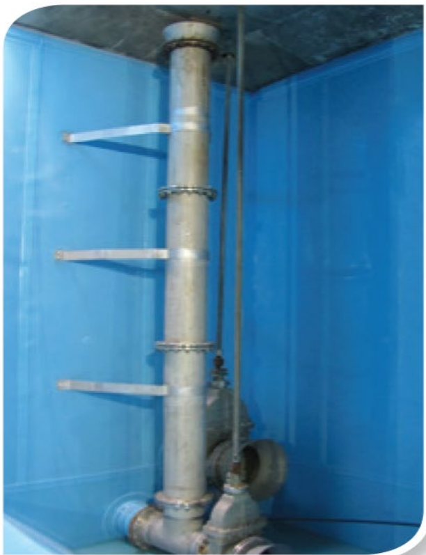
After installing collecting well
