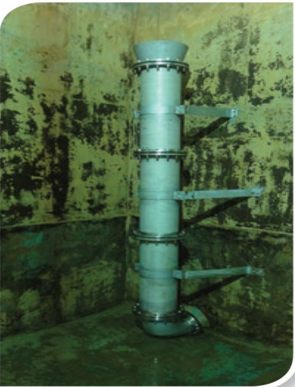
Before installing collecting well
