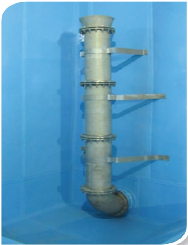
After installing collecting well
