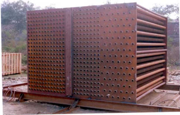
Recuperator in Pre-assembly Stage
